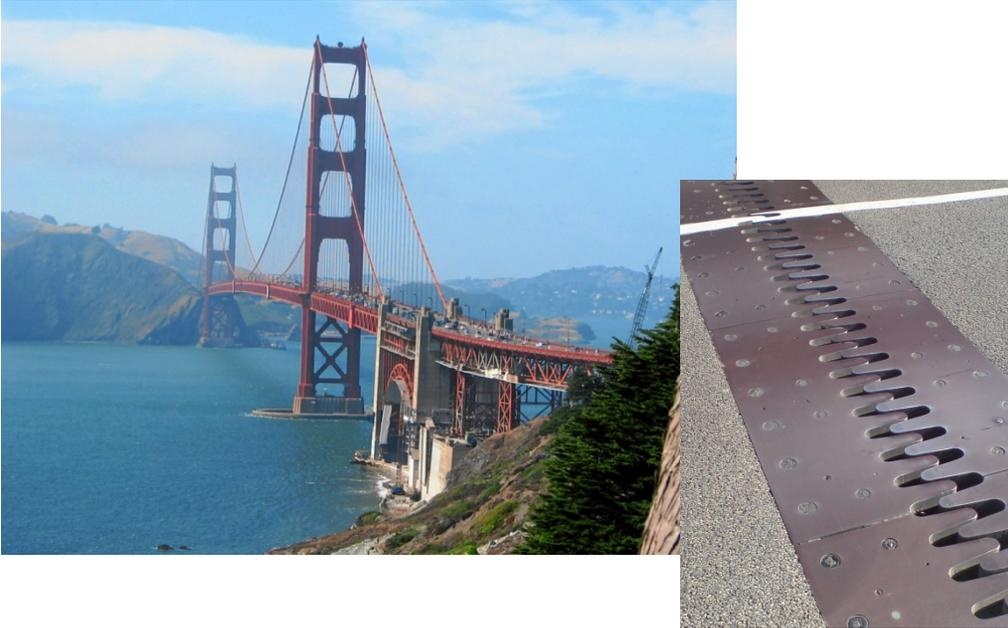
When engineers design roads and bridges, they include expansion joints at key locations. These joints are necessary for the structures to remain stable over time.
